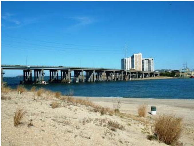
The twin replacement bridges will each feature a 53 foot eight-inch wide deck that will accommodate two lanes of traffic, with appropriate shoulders on each side and a multi-use path in each direction. The eastbound and westbound structures can accommodate three lanes of traffic in each direction in the future, if needed.
